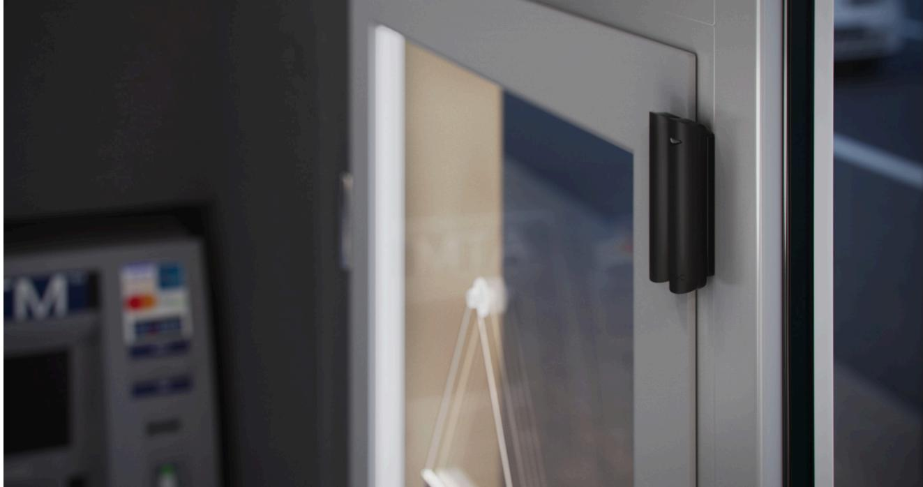
If the window has a ventilation mode, the detector should be installed on the upper part of the window. Otherwise, when the window is opened for ventilation, the detector gets closer to its own magnet and may perceive it as an attempt to mask it. To avoid false alarms, install the detector on the upper part of the window.
