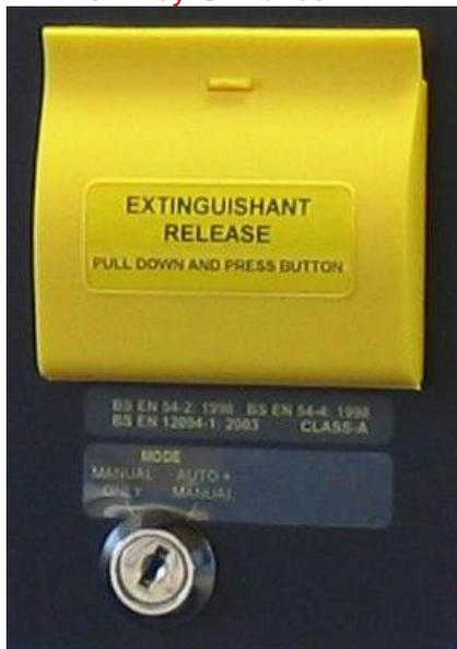
One key-switch is fitted to the panel.
